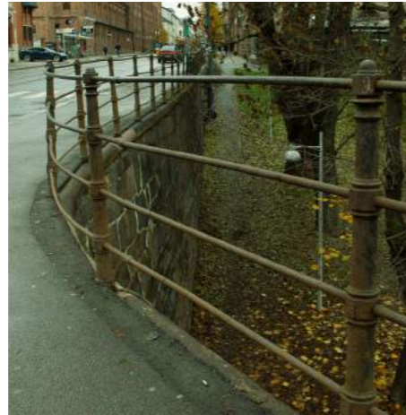
Parts of the railing can still be found today
