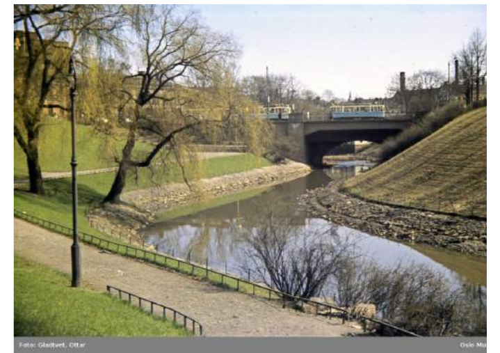
Before the underpass was built
